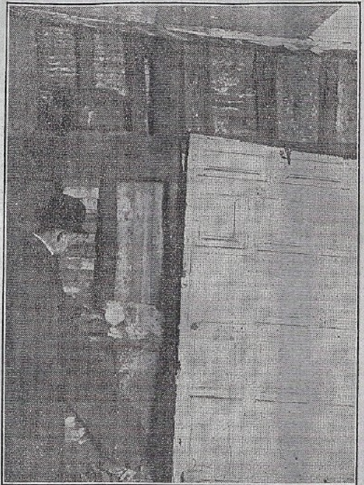
Picture gives some idea of the composition of the walls of an old house now being demolished in Butcher Row. Walls being brought to light through the removal of panelling show that the spaces between the beams were filled in with clay and straw.
