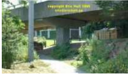
Illustration 3 - Medieval city wall demolished to make room for a flyover support – Photograph by Eric Hall July 2006
